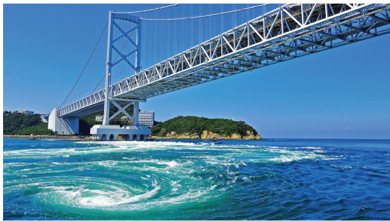
鸣门跨海大桥 Onaruto Bridge
