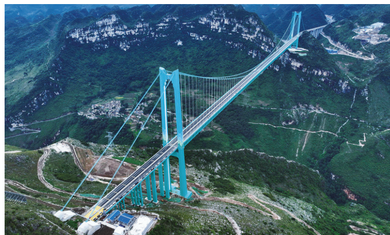
花江峡谷大桥 Huajiang Canyon Bridge
