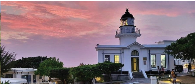
旗后灯塔 Qihou Lighthouse
